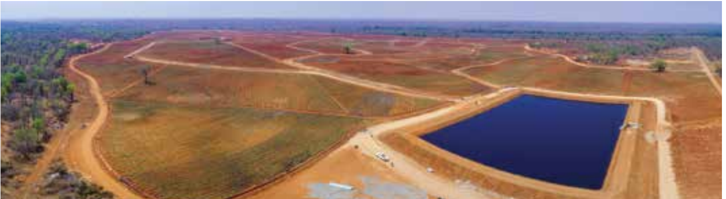
• Aerial view of Project Kilimanjaro
